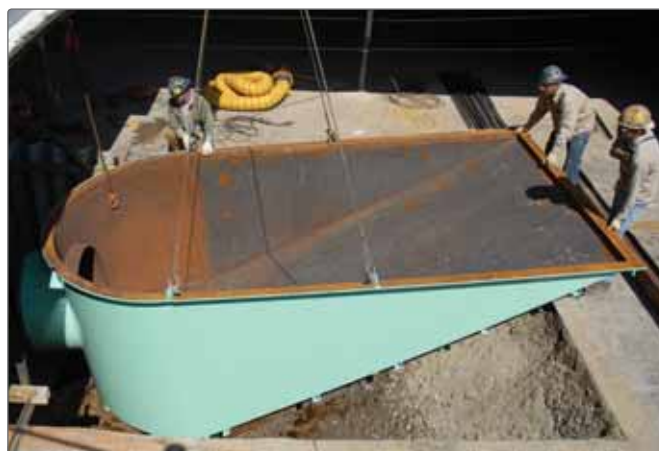
Tank bottom treatments such as drain dry sumps or mesa bottoms can have significant impacts on heel reduction.
