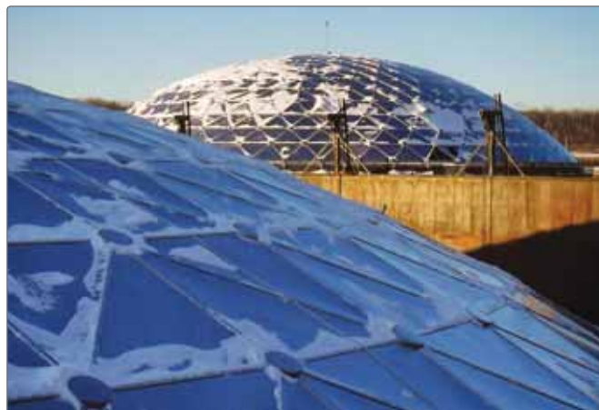
Aluminum domes offer several advantages, including superior corrosion resistance and positive impacts to both tank capacity and emissions mitigation.
